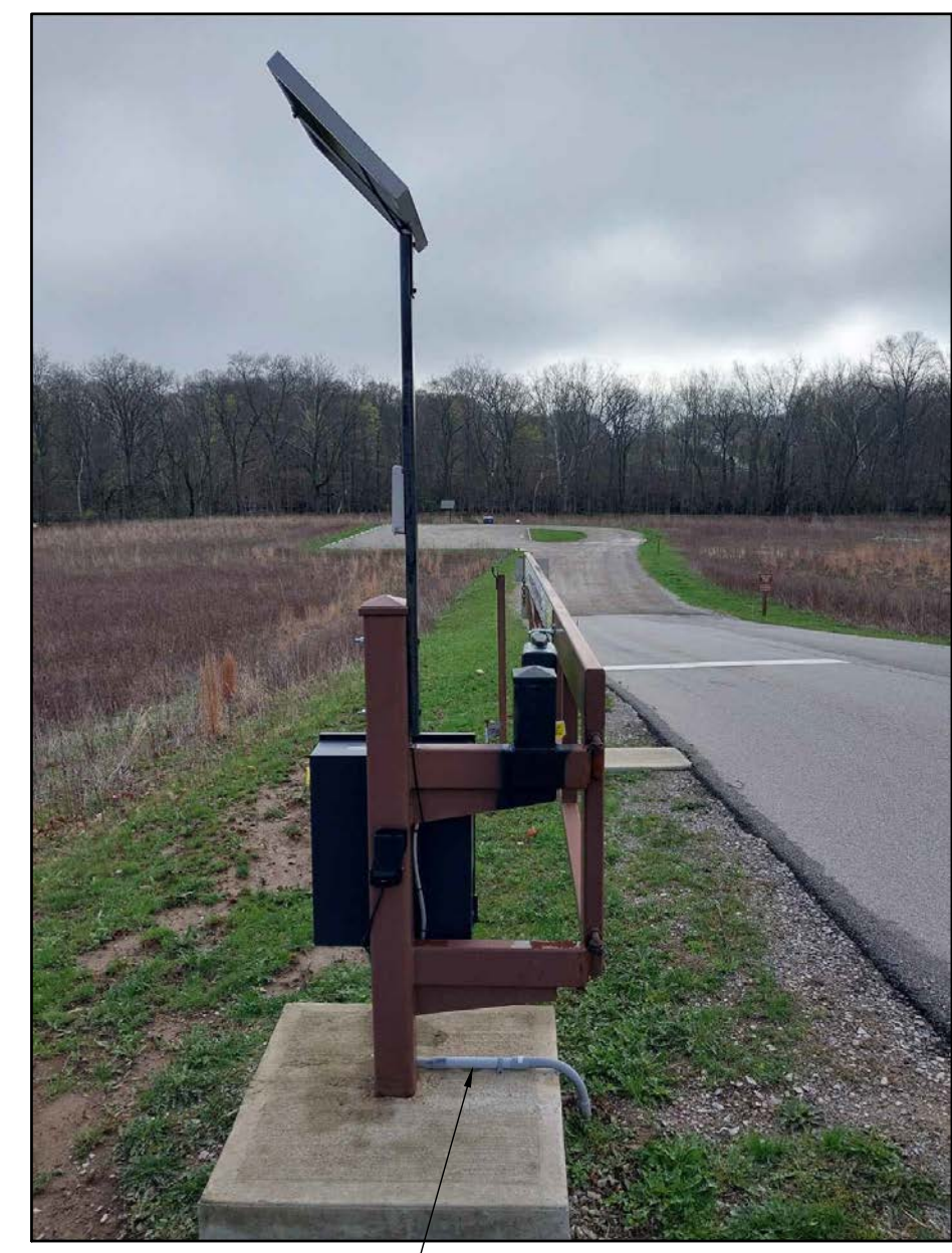
1" CONDUIT UNDER ROADWAY TO SECONDARY OPENER.
