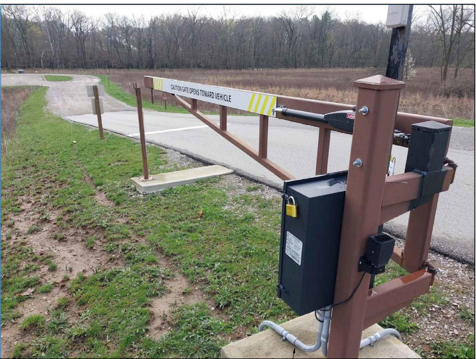
CONDUIT TO AUTOMATIC GATE OPENER EXIT SENSOR
